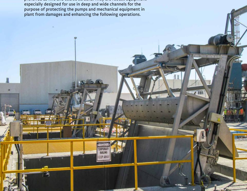
This type of screen can be easily mounted in any channel depth at an angle between 60° and 90°, generally preferred in deep channels due to its durable structure.
