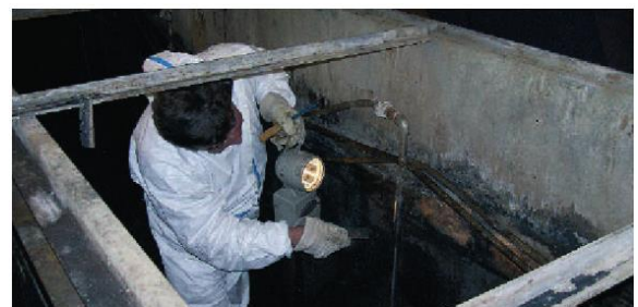
HUBER Refurbishing Service
