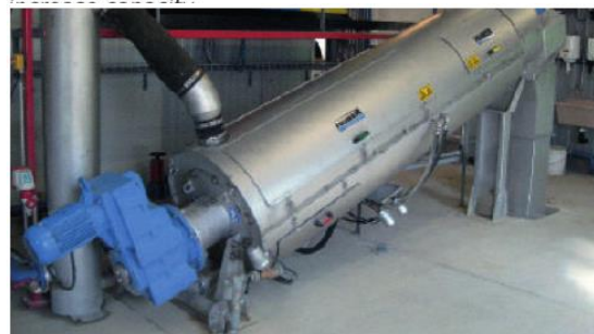
HUBER Screw Press S-PRESS: Specific power consumption < 0.01 kWh/kg DR
