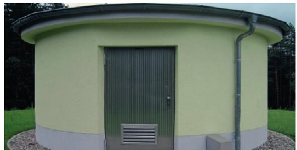
Drinking water reservoir with HUBER equipment
