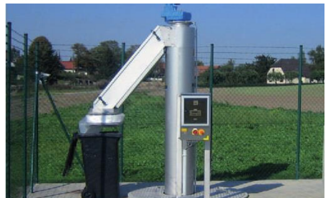
HUBER Pumping Stations Screen RoK4 with heating for outdoor installation
