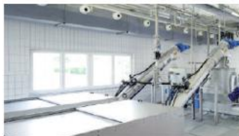
HUBER Rotary Drum Fine Screen ROTAMAT® Ro2 with up to 3 m screen basket diameter
