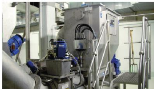
HUBER Wash Press WAP® HP: Pressure regulation guarantees continuously high solids content
