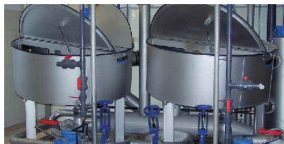
Installation of two units in parallel for WWTP sizes of up to 200,000 PE
