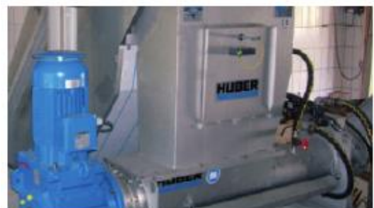
HUBER Wash Press WAP® installed behind a HUBER Fine Screen STEP SCREEN®
