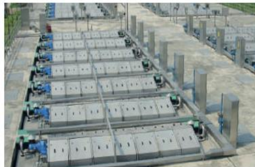
HUBER Disc Filter RoDisc® with up to 35 discs in one unit
