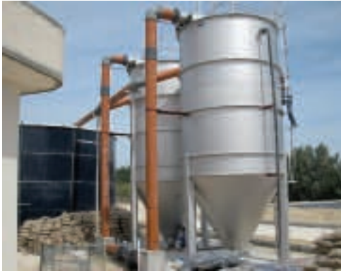
CONTIFLOW® Sandfilter CFSF, stainless steel tank design
