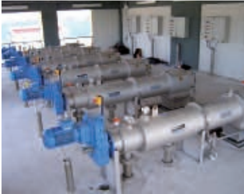
STRAINPRESS® – continuous pressurised coarse material separation
