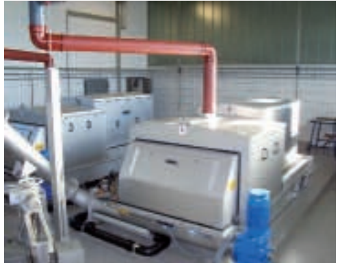
Compact Curved Bar Screen CurveMax® for reliable separation of solids from wastewater
