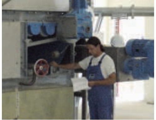
HUBER repair service
