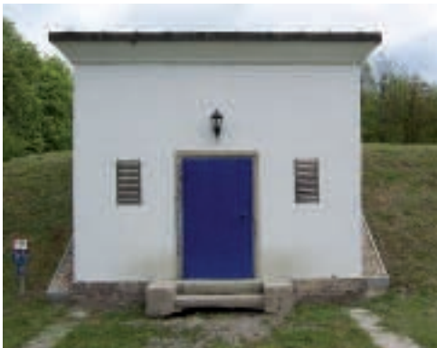
Drinking water reservoir with HUBER equipment
