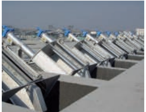
ROTAMAT® Fine Screen Ro 1 for channel or tank installation
