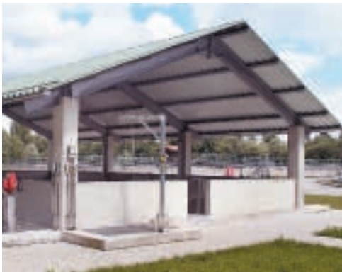
CONTIFLOW® Sandfilter, concrete tank design
